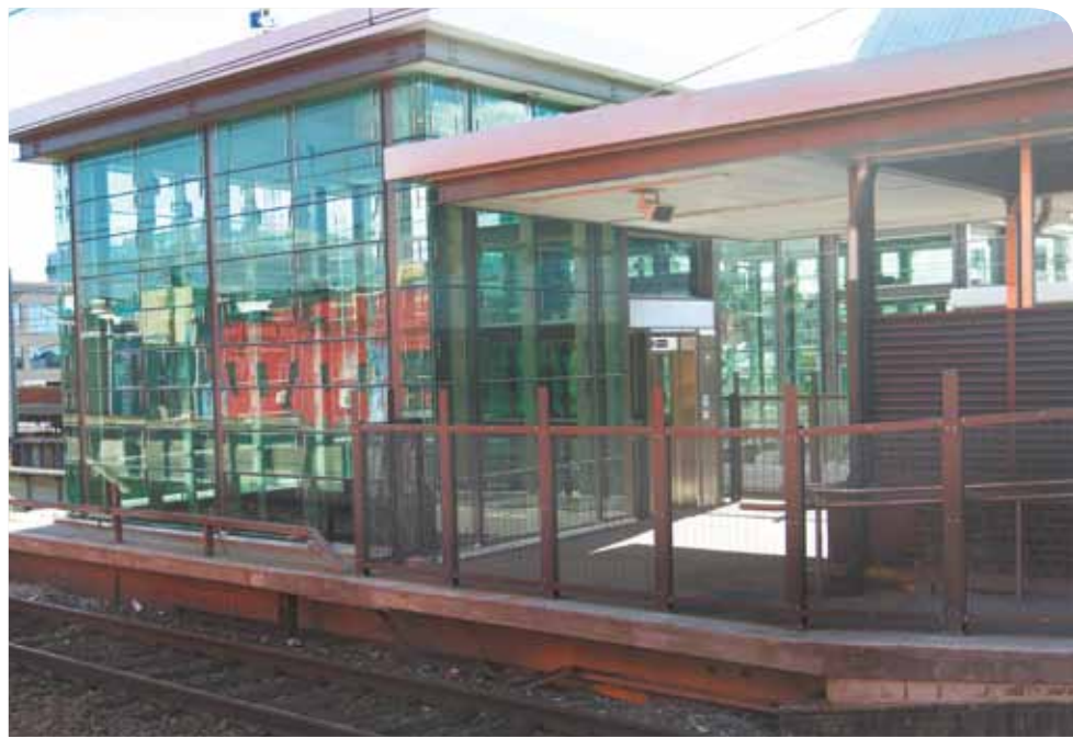
Burwood Station's recently-completed upgrade includes four new lifts
